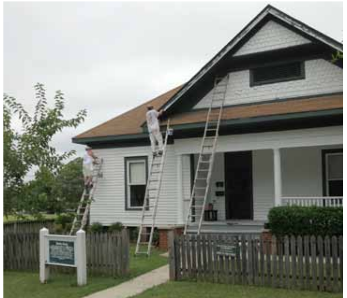
T.C. Roll & Son at work on Duncan House. Photograph August 2013 by Marjorie White.
