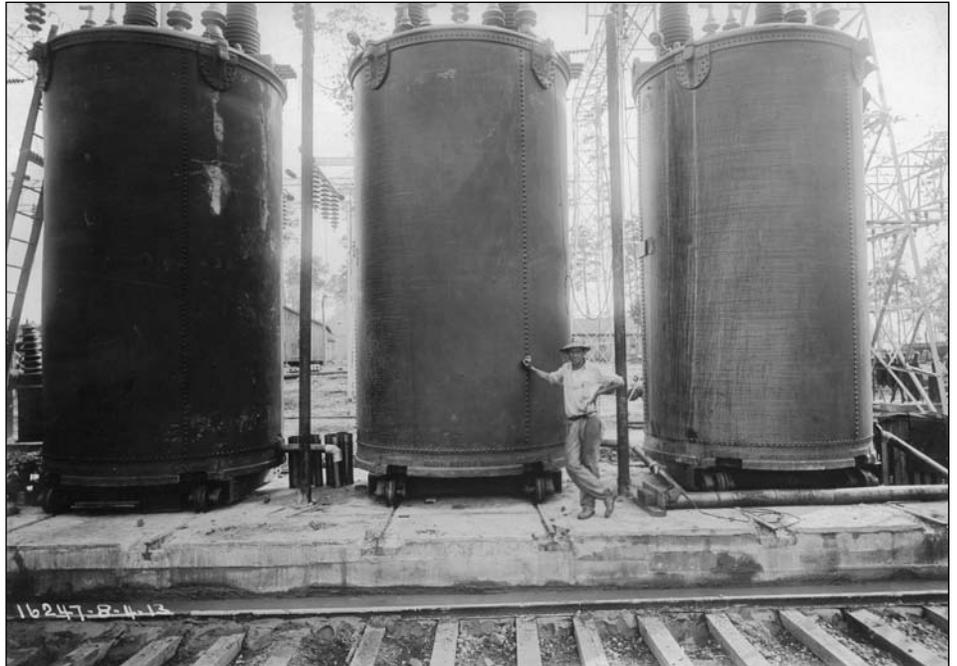
*Transformers at a Substation, Gadsden, Alabama, August 4, 1913. Courtesy Alabama Power Company Archives. In these tanks high voltage electricity generated at the Lay Dam on the Coosa River was transformed into lower voltage current. The "stepped down" electrical current is sent to distribution stations throughout the service area for delivery to individual customers.*
