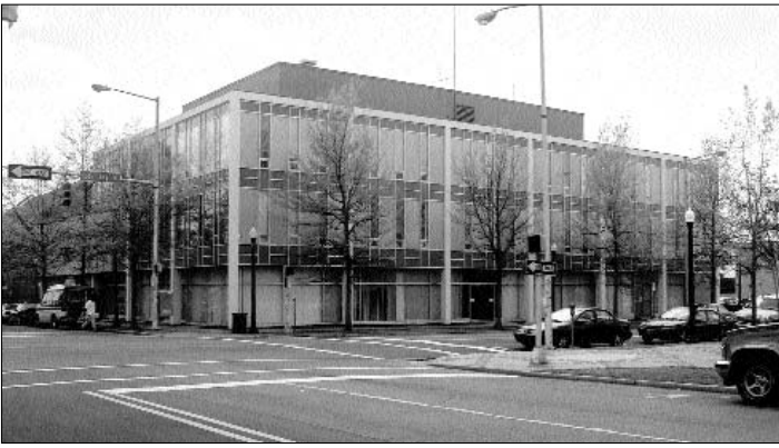
A. G. Gaston Building & L. R. Hall Auditorium, 1959 Fifth Avenue North at 16th Street
