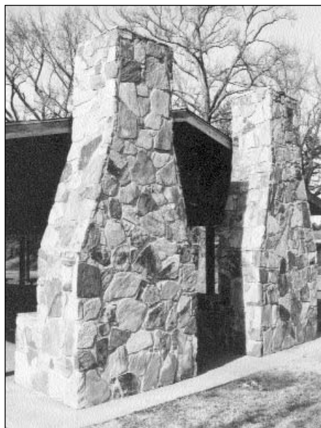
Twin Bar-B-Que Chimneys, built as ancient iron furnaces by masons employed by the C.P.A., 1933, Green Springs Park, Adam Colbert
